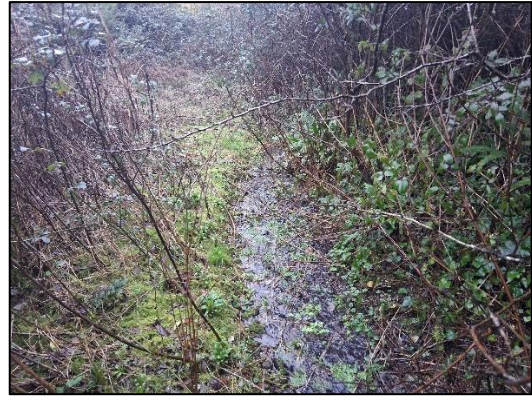
Plate 2-7 Unmapped watercourse flowing east, from the culvert.
